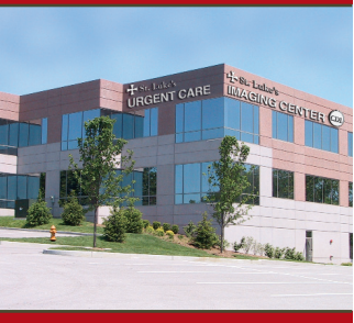
WingHaven® Medical Building
